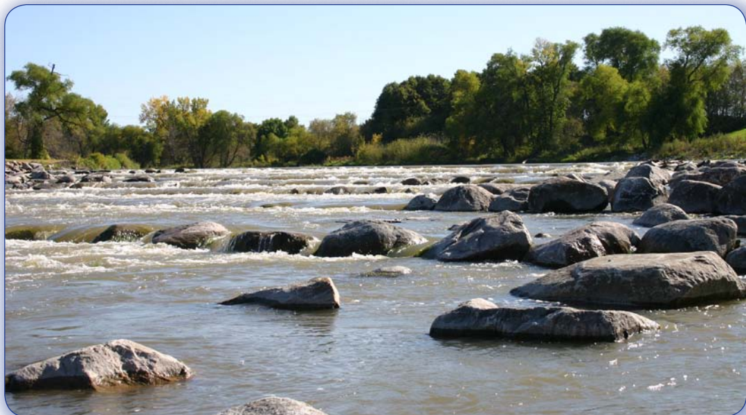
Figure 102. Photo showing completed Crookston Rapids.
