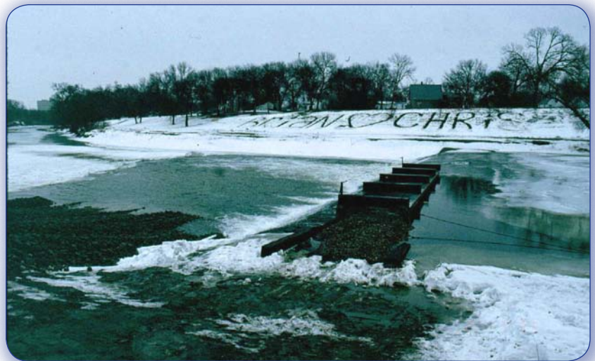
Figure 72. Temporary partial diversion using steel I-beams placed on the dam crest.
