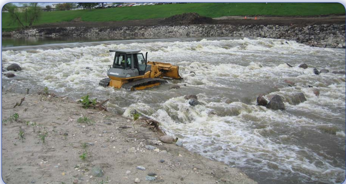
Figure 100. Grading of the fieldstone base with a bulldozer in May, 2005.
