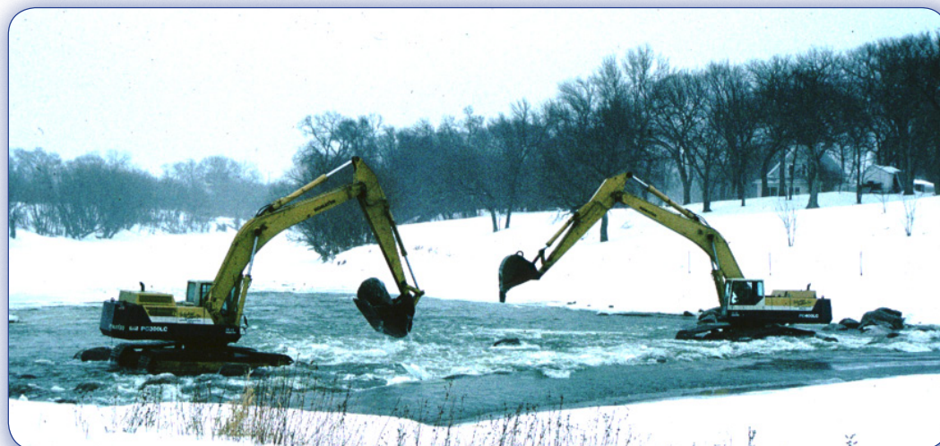
Figure 74. Two excavators using a bucket-brigade technique for placing weir stones.
