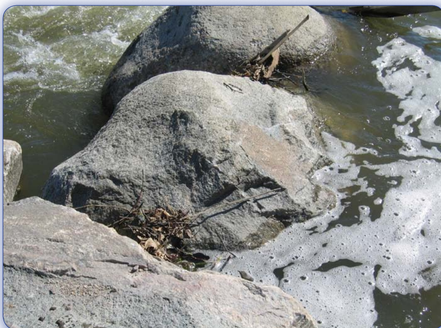
Figure 55. Leaves and woody debris sealing void in a rock rapids fishway.
